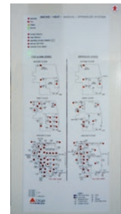
Typical purpose-built indicating boards: Left Fire fan indicator panel Right Network zone index
